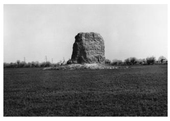
Fig. 14 Stupa of Zurmala: It is said to have been constructed during the reign of King Kanishka. As calculated by Pugachenkova, 1.2 million sundried bricks were used in its construction.
