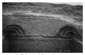
Fig. 24 Squinch arch. Traces of circular dome
